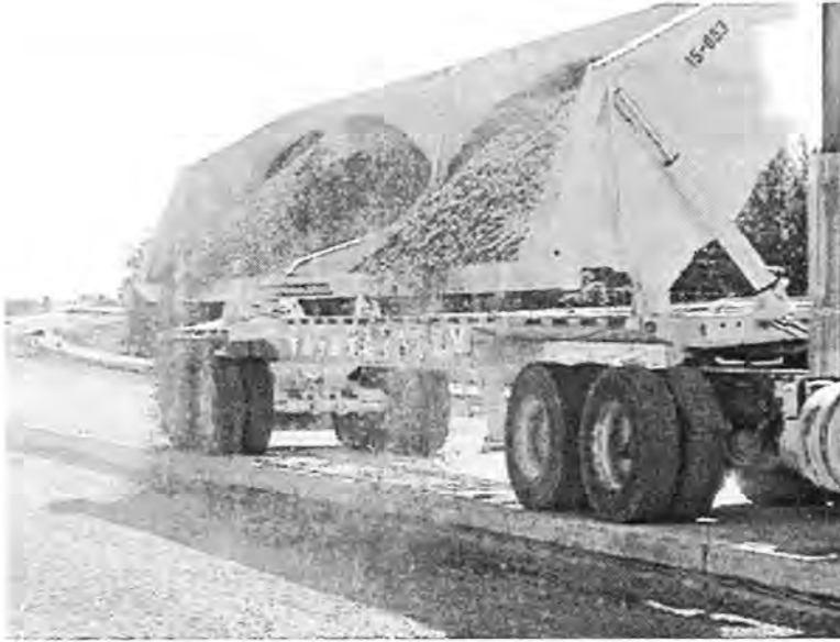
Figure 52. Another method of dumping the aggregate
