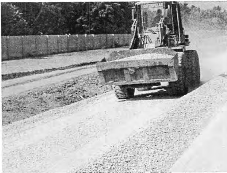
Figure 54. Bucket loader removing excess aggregate
