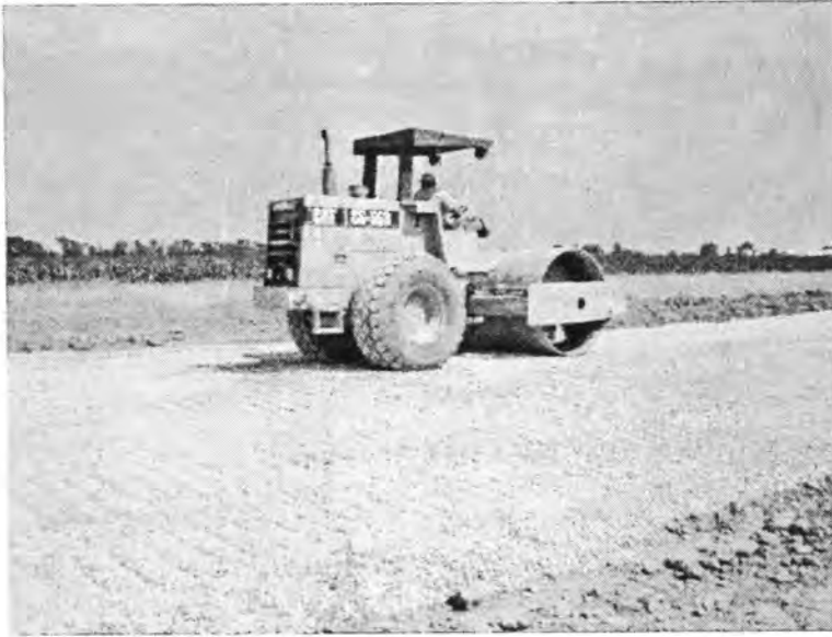
Figure 37 Initial Compaction using 563 CAT Roller
