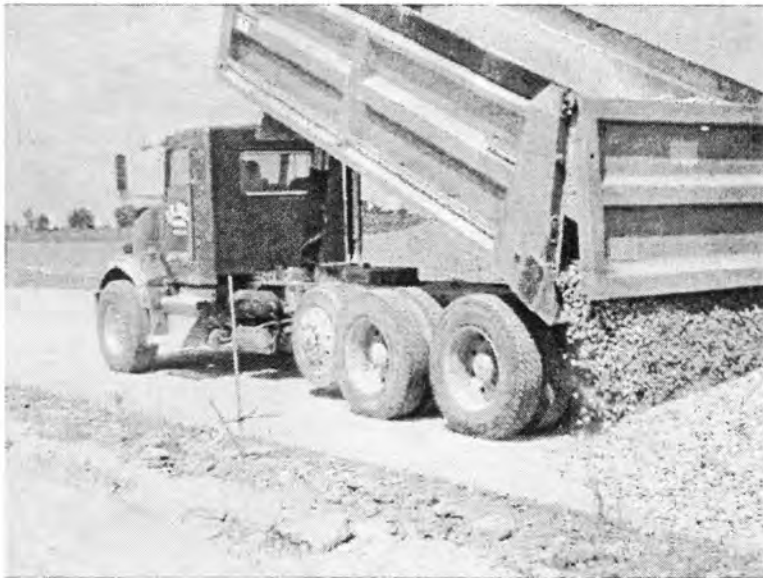
Figure 35. Dumping of aggregate on subgrade
