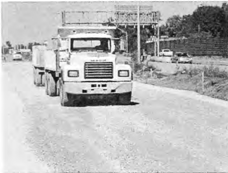
Figure 49. Trucks moving on base for placing the aggregate
