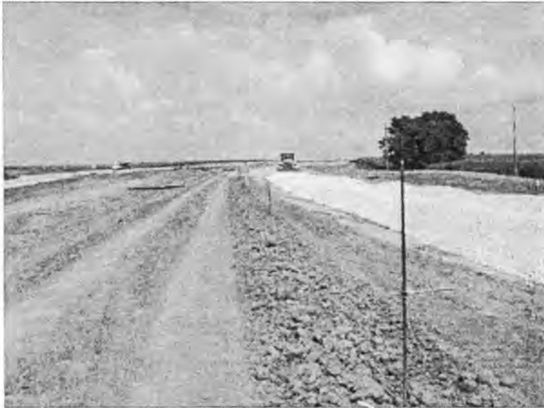
Figure 44. Haul way used by the trucks to transport the aggregate
