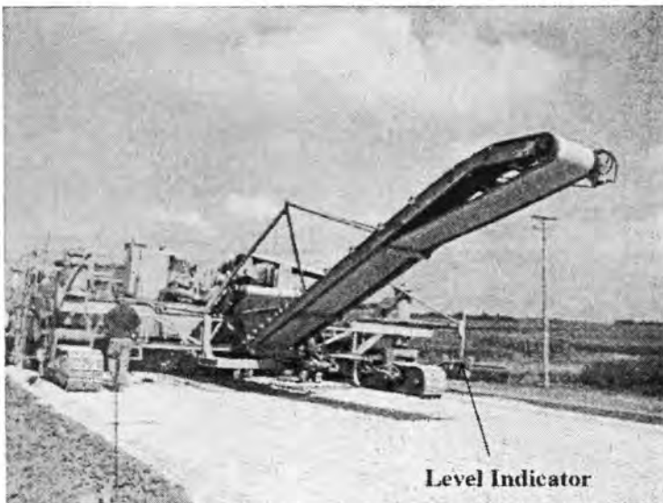
Figure 46. Final trimming process using TR 500 trimmer
