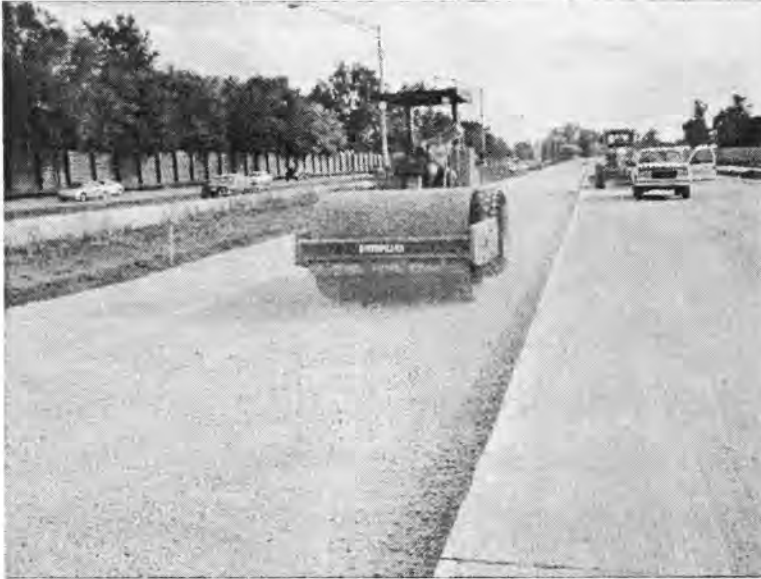
Figure 55. Roller used for final compaction
