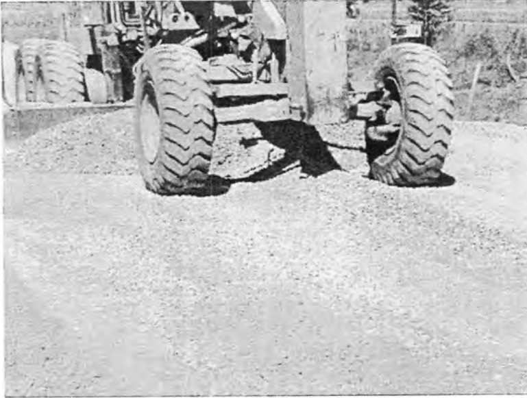
Figure 53. Spreading and trimming of aggregate
