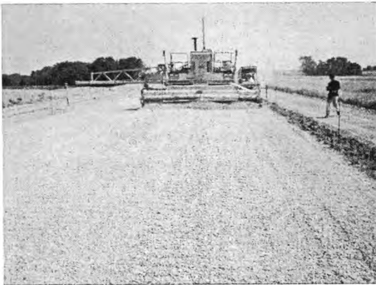
Figure 38. Final trimming using 9500 Gomaco
