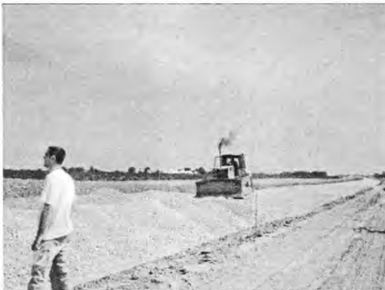
Figure 36. Spreading of aggregate piles using D6XL dozer
