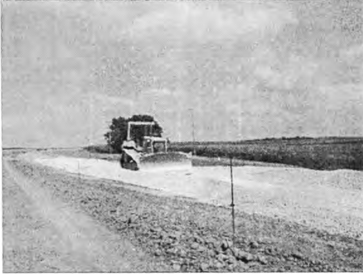
Figure 45. Spreading of aggregates using a D6XL dozer
