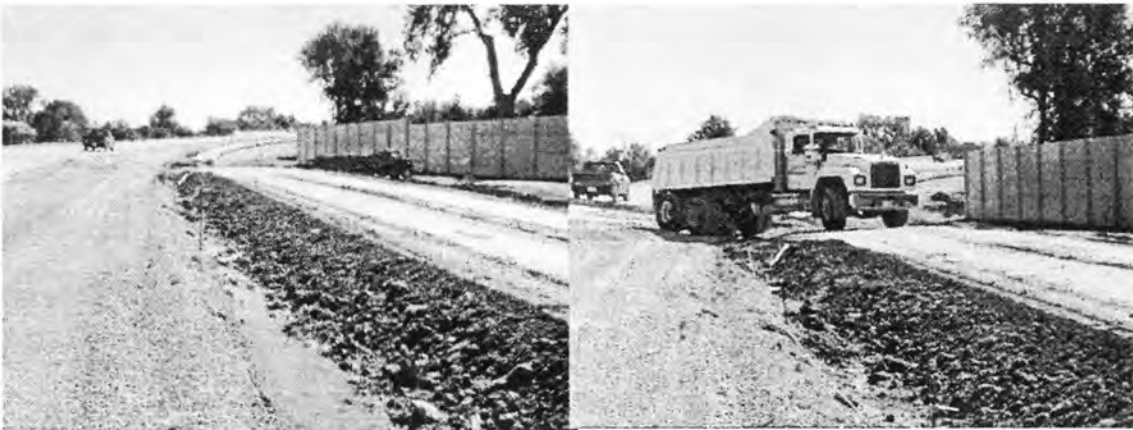
Figure 51. Trucks using haul way on their way back to the quarry
