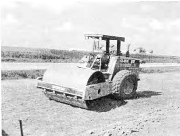
Figure 48. Roller used for final compaction
