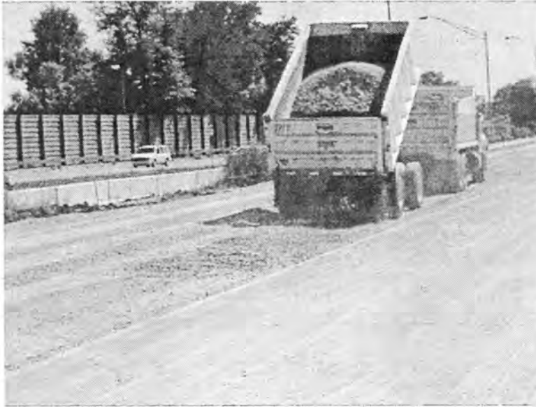
Figure 50. Dumping of aggregates from the truck
