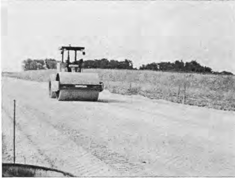
Figure 41. Final compaction using 563 CAT roller
